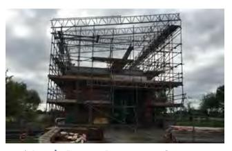
North Drain Pumping Station Replaced 50-year-old leaking concrete roof with lightweight new roof, along with other
