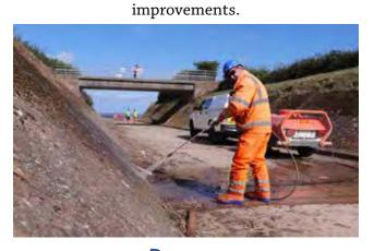
**Dunster**Repairs to the River Avill Flood Relief Channel and erosion protection at Gallox Bridge.
